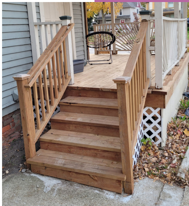
Porch repairs done through an Alliance Catholic Foundation grant. (Photo: Friends of the Master)
